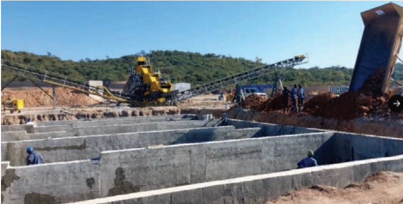
c) Building the settling ponds
